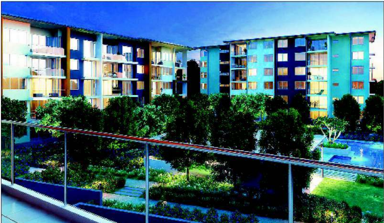
The Rayjon Group's Island Grove project is one of a raft of developments being rolled out this year on the Gold Coast's north shore
